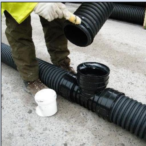
**Step 4- Push the fitting onto the end of the Pipe with the rubber seal fitted.**
