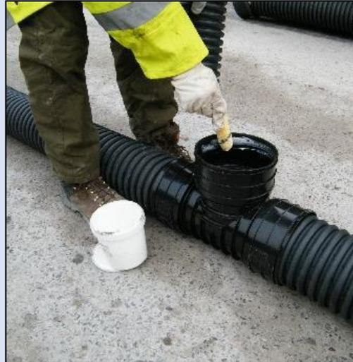
**Step 3- Apply Pipe Lubricant to circumference of the rubber seal as shown.**
