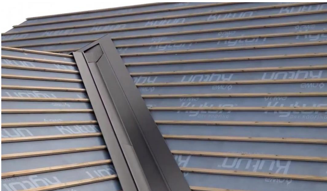
Valley Trough and Trim installed
