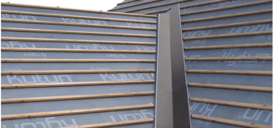
Valley Trough installed.
