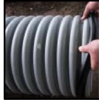
Putting on the sealing ring.
