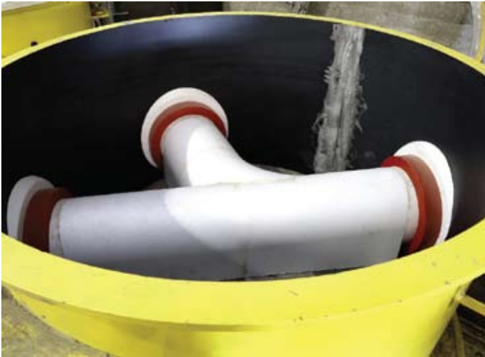
Installation of F910 Connection Seal
